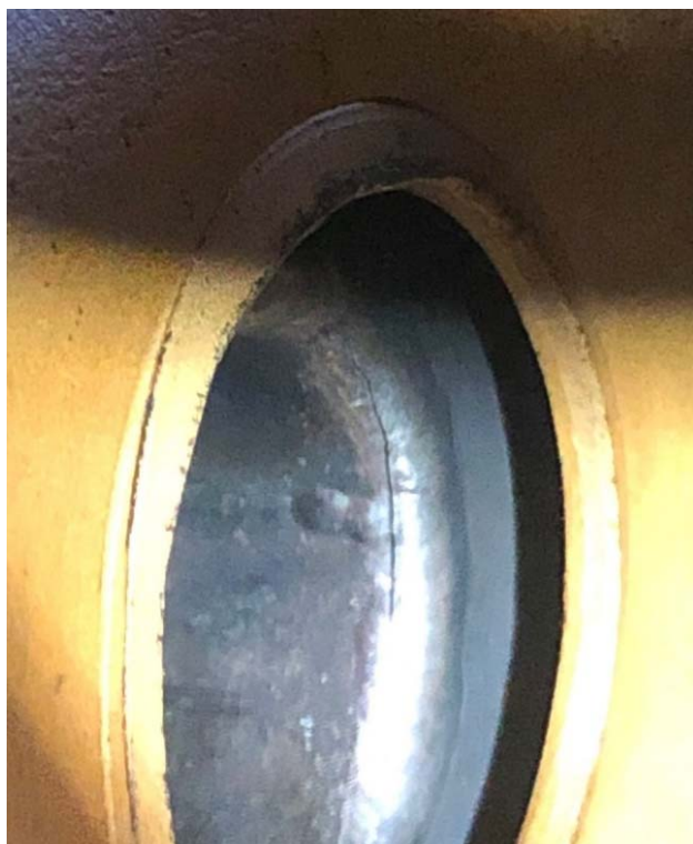
Fig 1. Hanger with Weld Crack.
